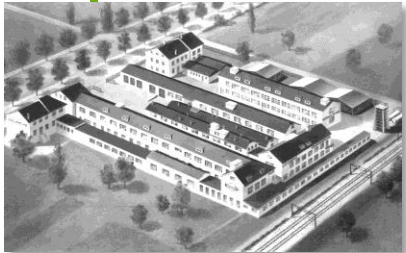
Leclanché SA is founded in Yverdon-Les-Bains, Switzerland.
